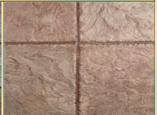
18" x 18" Belgium Slate Tile Stamped Concrete Pattern
